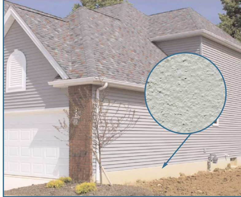
Horizon Coarse Coat (shown in photo above) provides a durable, textured topcoat that repels moisture and gives exposed foundation an attractive, finished look.
